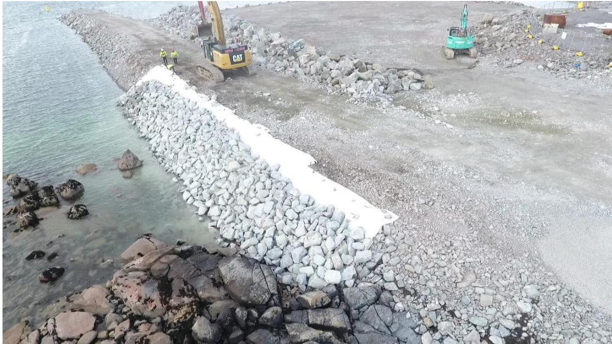
Plate 1-6. Construction of rock armour for the revetment (underlaid with geotextile).
