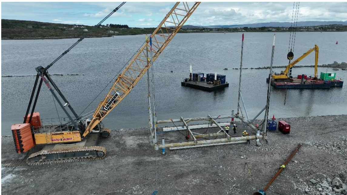
Plate 1-2. Bespoke frame used to accurately lower the quay wall foundation beams in place.
