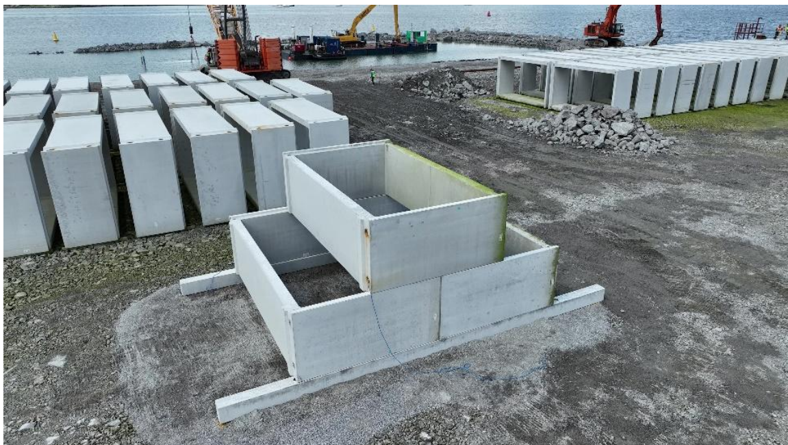
Plate 1-4. Mock-up arrangement of concrete box caissons on precast concrete ground beams.
