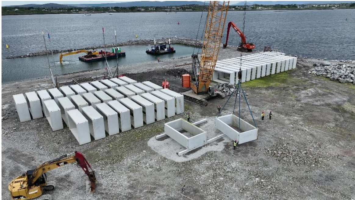
Plate 1-1. Concrete caisson boxes (7 x 4 x 2 metres) being placed on precast concrete foundation beams during onshore trials.
