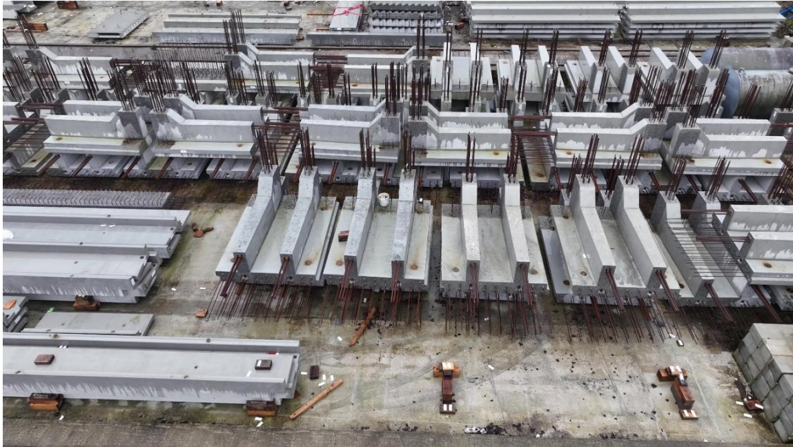
Plate 1-5. Precast wall sections to be placed on top of uppermost row of box caissons.
