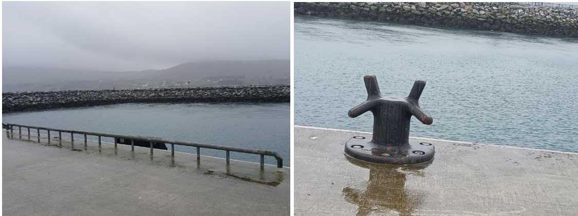
Plate 1-8. Security/Safety facilities to be installed along the quay wall – toe rail (right), and bollard (left).
