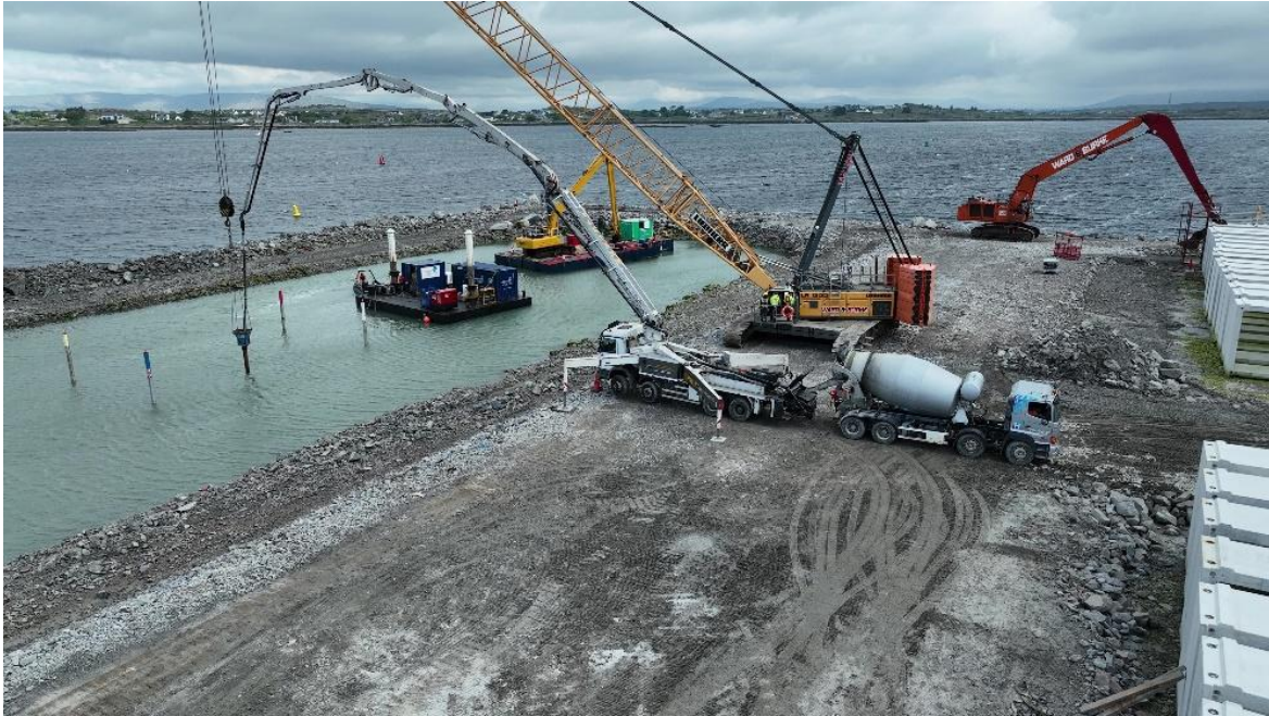
Plate 1-3. Anti-washout liquid concrete being delivered via Tremie Pipe and directed by underwater divers to surround and hold the foundation beams in place.
